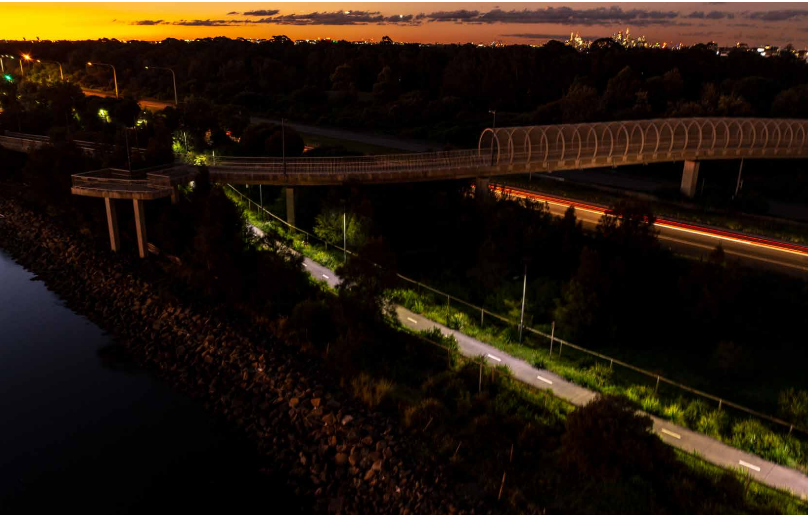
Above: Excellent uniformity and lux levels along the 2km pathway stretching around the shore at Port Botany opposite the freight terminal and Sydney Airport. Fittings were installed at 5.5m and spaced every 20m . The lighting plan met standard AS1158.3.1:2020 Table 3.4 PP3 for Pathways and Cycleways.. Below: SOLO 160W/130Ah solar engine coupled with Mako area light programmed to 20W (half the maximum output) to achieve the required light levels while providing autonomy of 4.5 days on a full charge.
